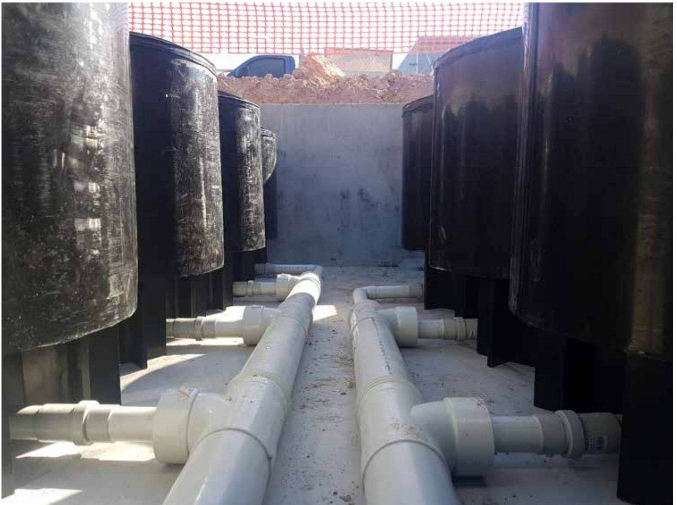
Figure 2. SPEL Filter install
