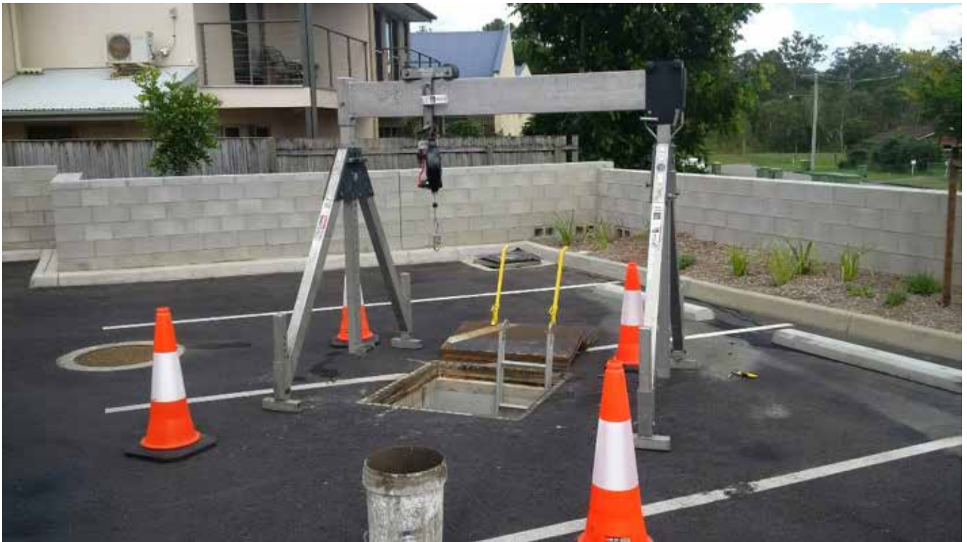
Figure 4. SPEL Filter install set-up
